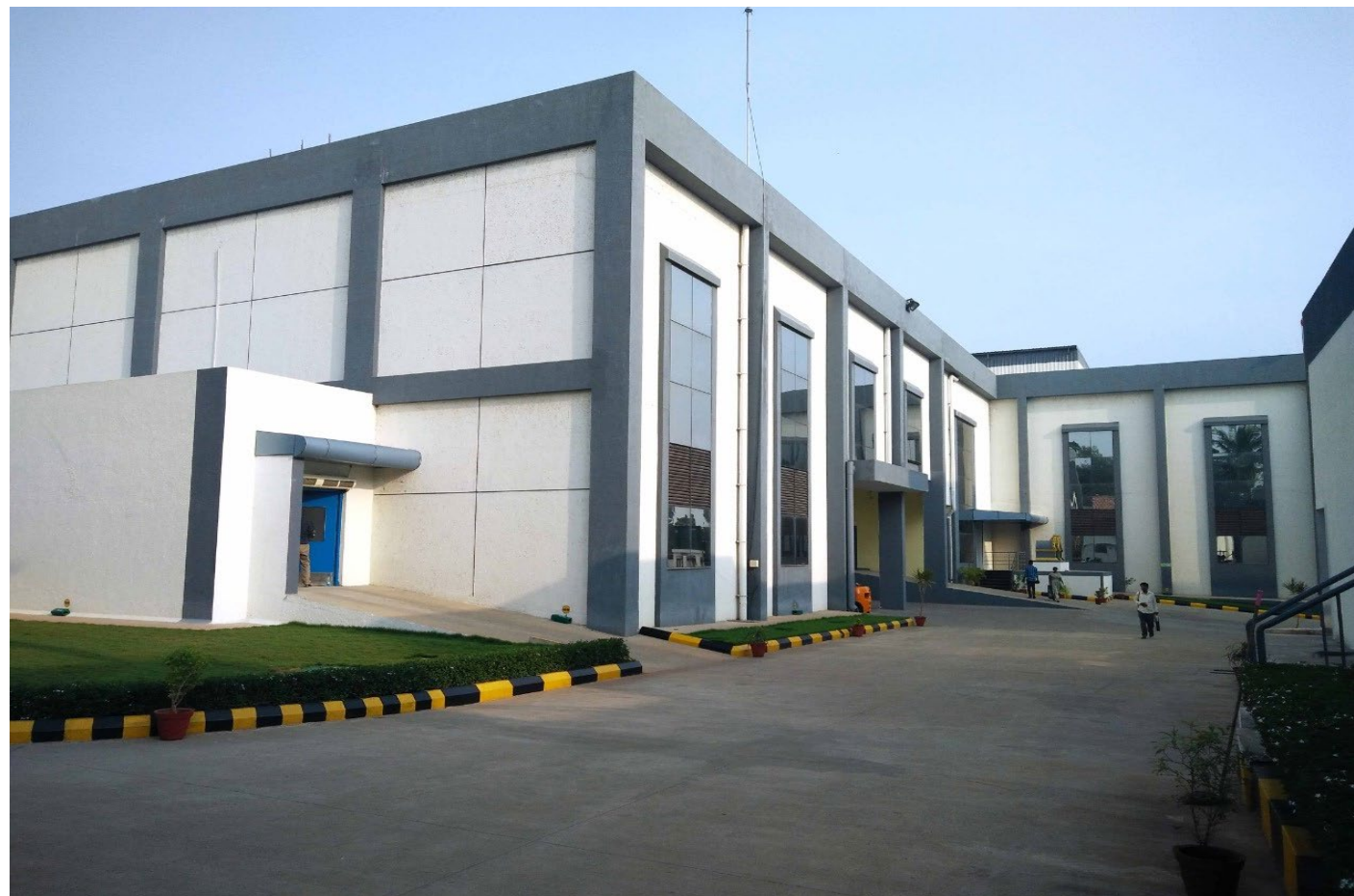
CP-I plant at Suthukeny, Puducherry
