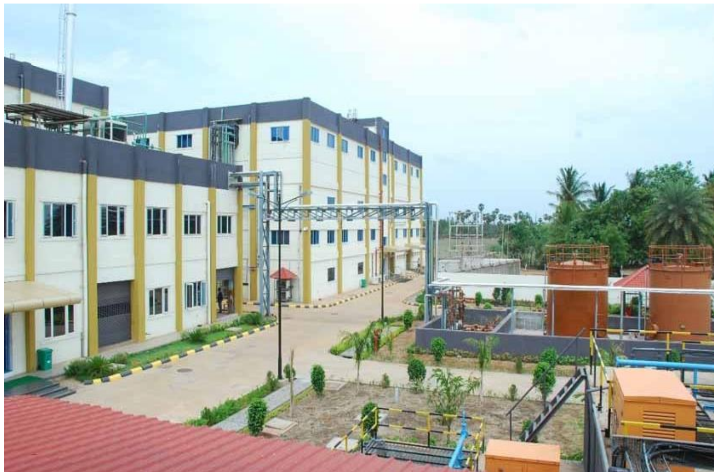
CP-IV plant at Gummidipoondi, Chennai
