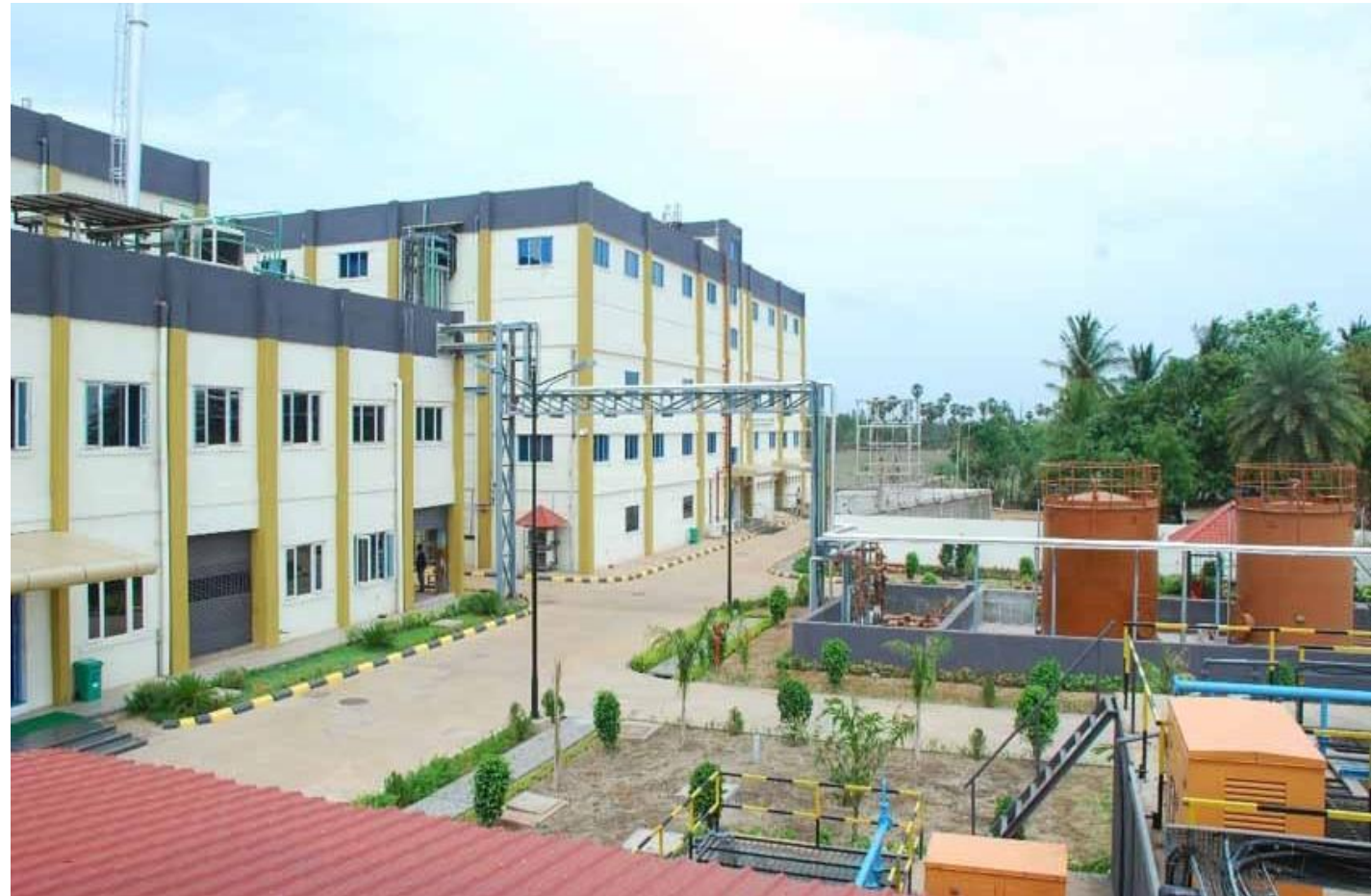
CP-IV plant at Gummidipoondi, Chennai
