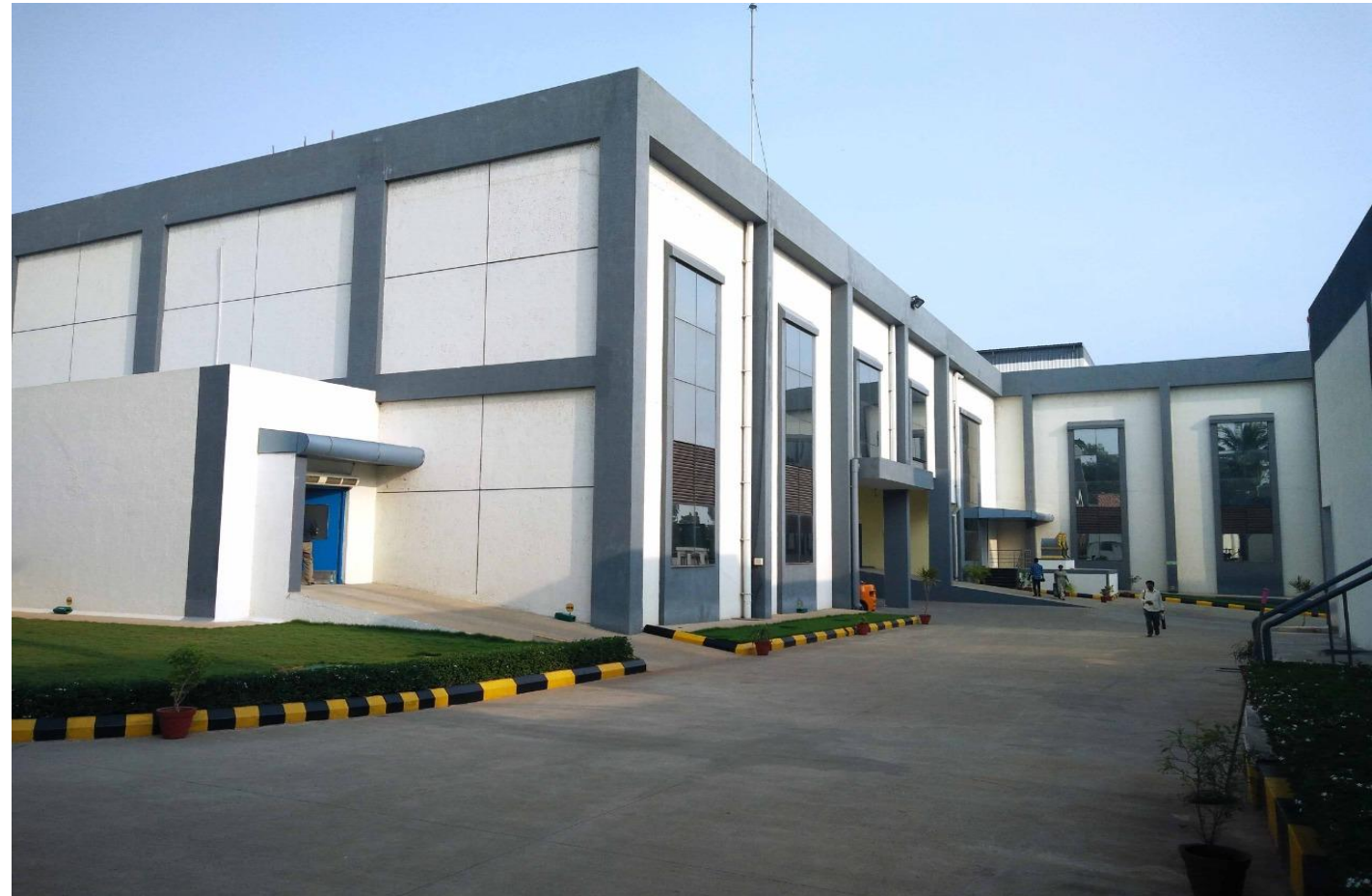
CP-I plant at Suthukeny, Puducherry
