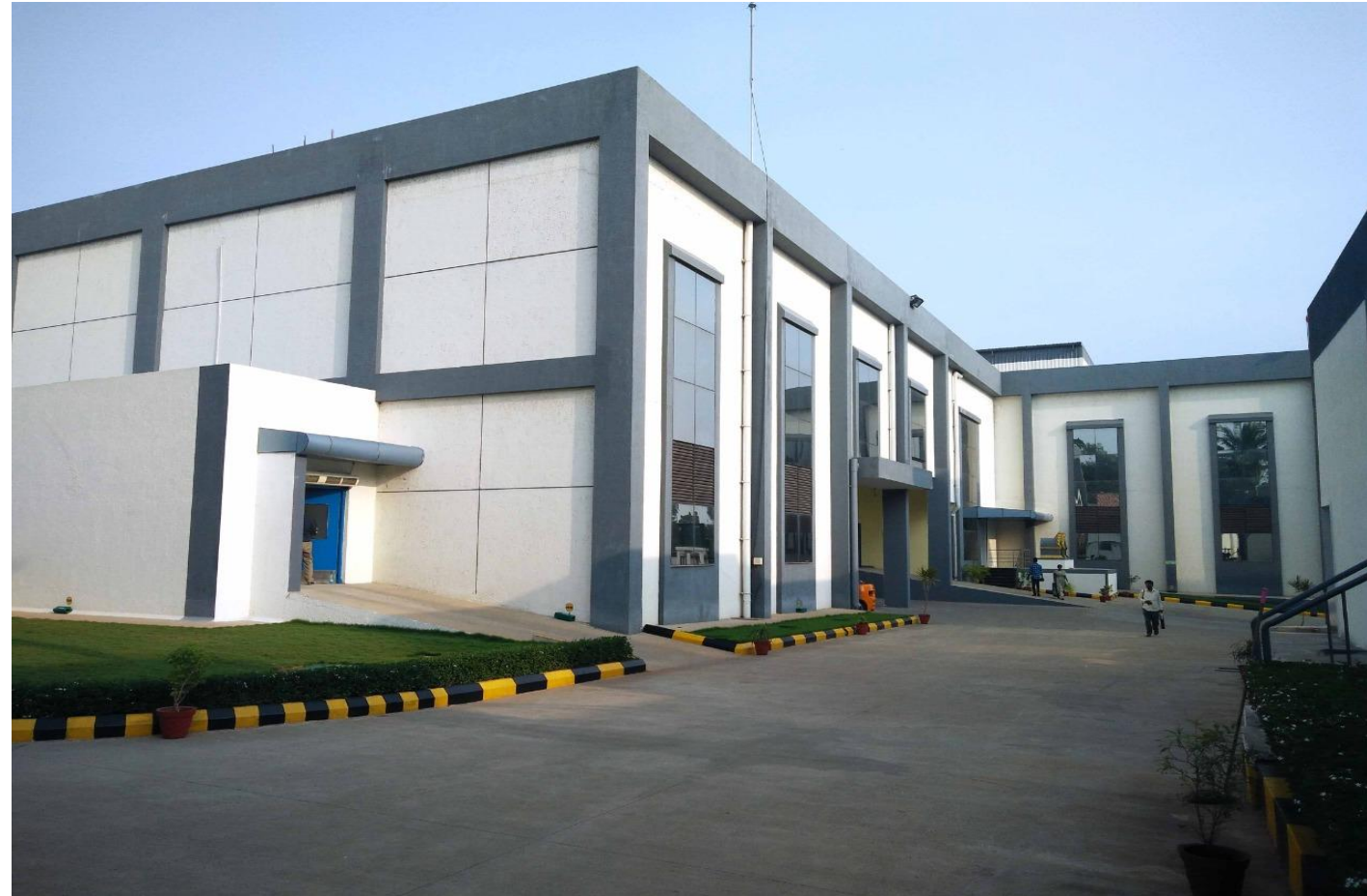
CP-I plant at Suthukeny, Puducherry
